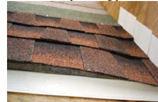
Step 7 ^ Continue by installing a starter course & shingles with a 1/2" to 1" overhang at the eaves edge. SmartVent End Caps are Patent Pending in the USPTO.
