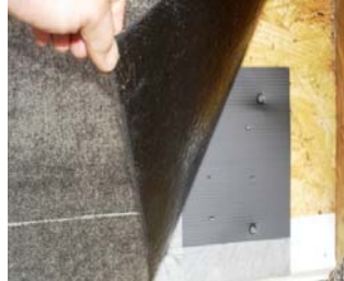
Step 4 ^ Install ice shield over SmartVent.
