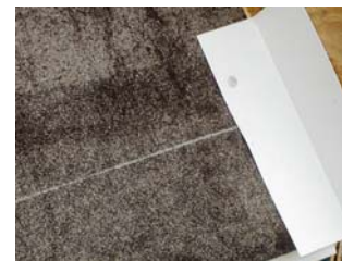
Step 6 ^ Install wall step flashing per code.
